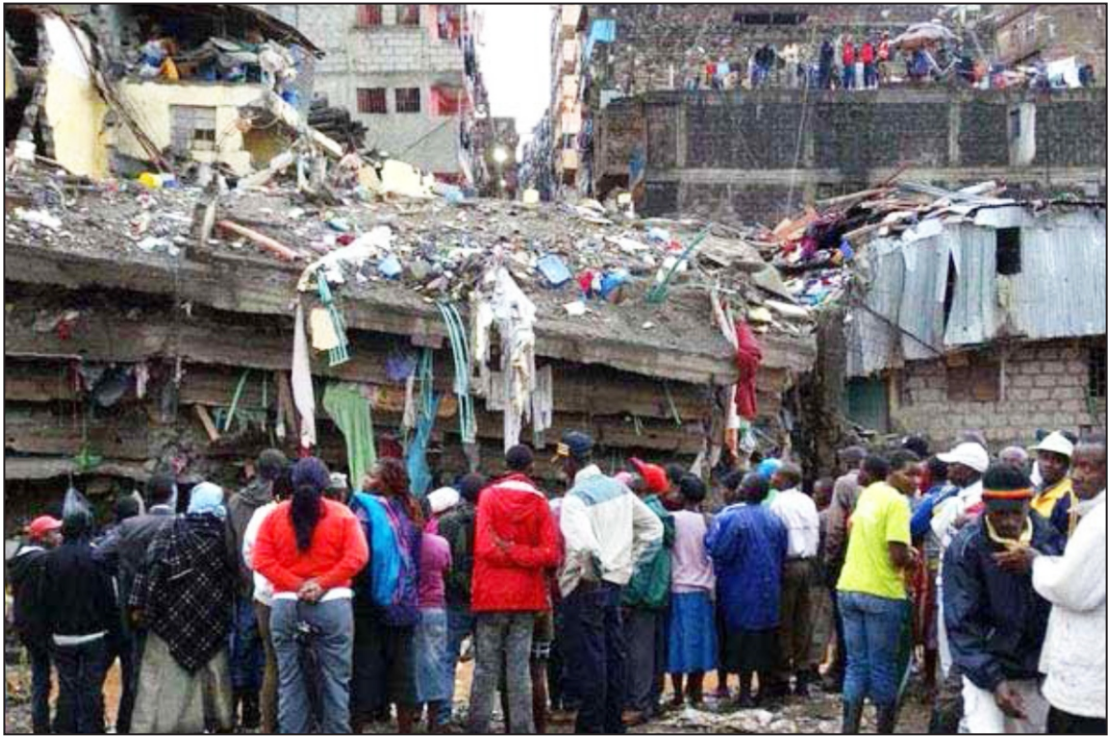
Figure 6.2: Collapse of residential building in Huruma, Nairobi County in April, 2014
