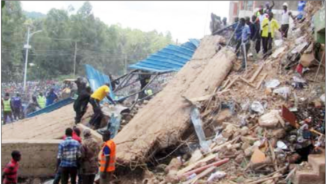
Figure 6.4: Collapse of Residential Development on Plot. N/B/Bobura/3546 in Mwembe Town, Kisii County in October, 2014
